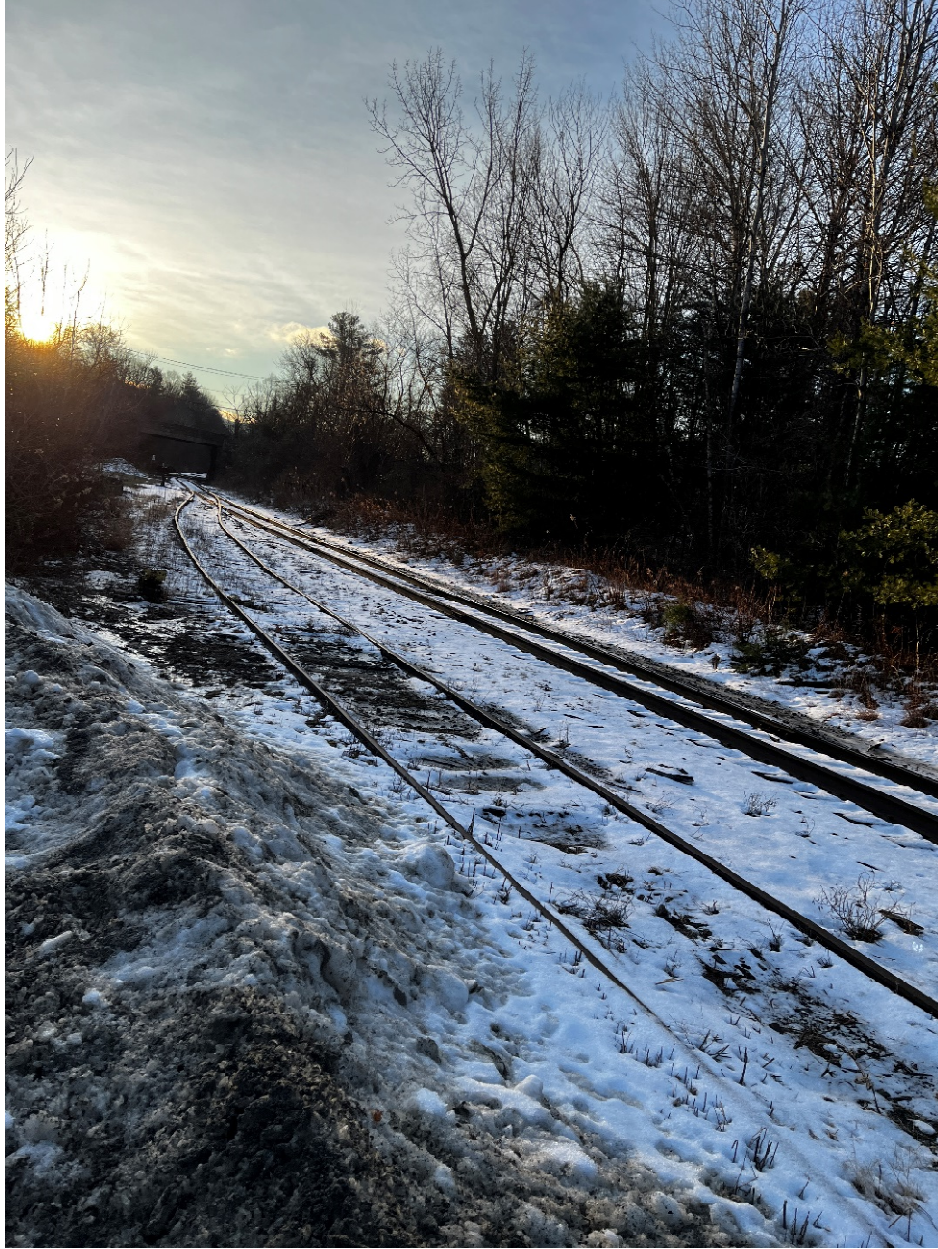
Approximately 0.47 miles of railroad siding adjacent to Industrial Drive in Pittsfield, north of Reach 6.
